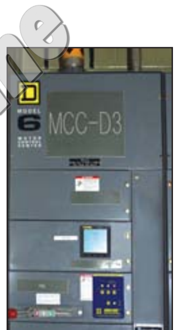
The PowerLogic meter continuously logs power usage, allowing for complete analysis that will lead to energy savings. The SurgeLogic meter protects equipment from surges, helping protect reliability.
